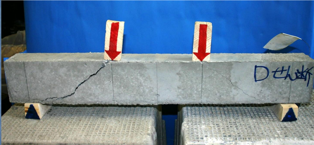
せん断破壊 shear failure
